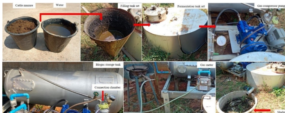
Figure 4. Composition of the biogas production prototype installed in the community field
